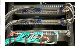
1U spacing between switches for proper cable routing
